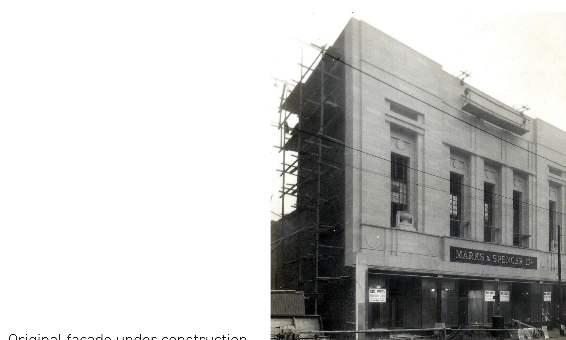
Original facade under construction
